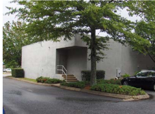
View of Rear of Subject Property
